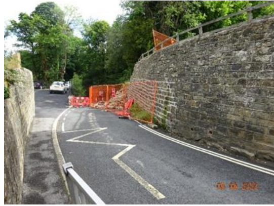
View look north along the street
